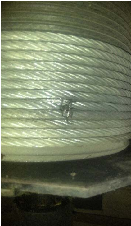
DAMAGED CABLE ON CLANCY MOTOR 1,
