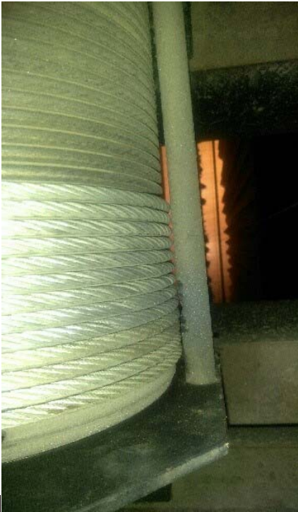
RUBBING CABLES ON DRUMSHAFTS
