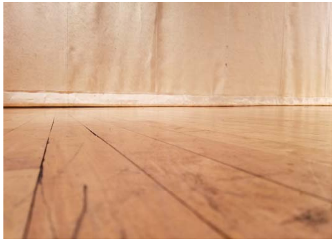
UNSEATED FIRE CURTAIN
