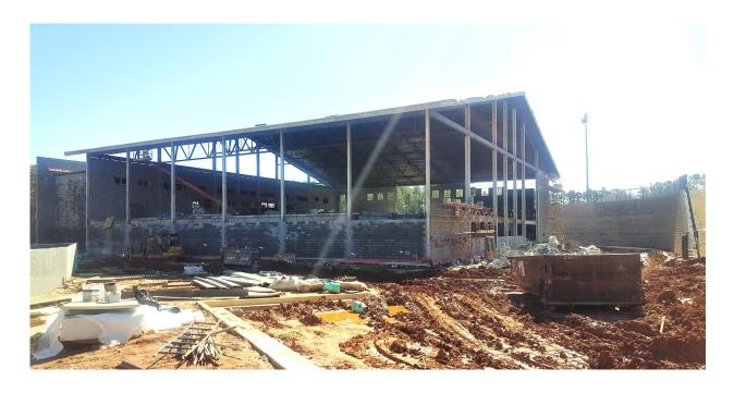
Riverdale High School's new Competition Gym continues to make forward progress. Steel erection has started and is complete with block and brick installation ongoing. Concur-
