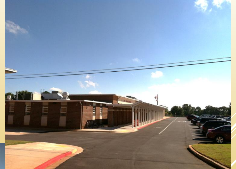
BABB MIDDLE YEAR COMPLETED: 2013 CONTRACTOR: BOWEN & WATSON ARCHITECT: MANLEY SPANGLER SMITH COST: $5,671,000
